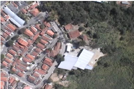
Figure 11 - Original Image Captured by the UAV.
